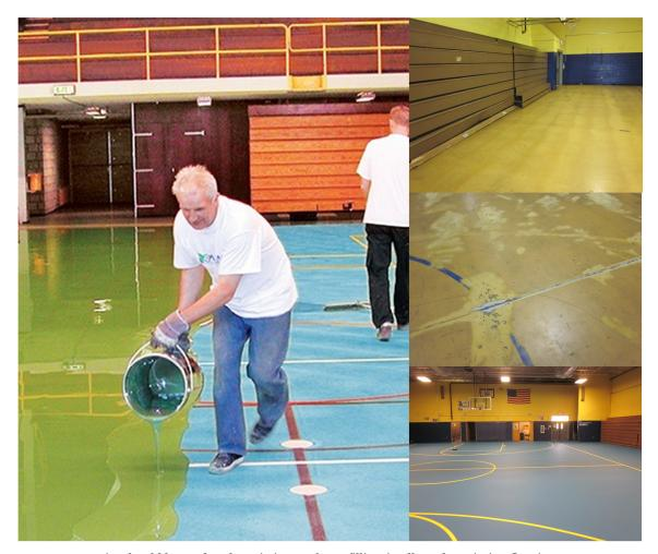
Repairs should be made t the existing surface—filling-in all cracks, missing flooring, and loose areas. Thoroughly clean the existing surface to remove and contaminates and waxes. Lightly sand/screen the cleaned existing surface to ensure proper bonding. Pour the new RT 210 resin, color coat , and game line, the previous exhausted surface looks and plays like new.
