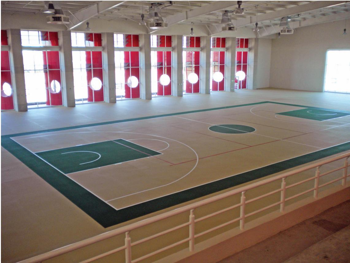
The MF systems are a dual durometer multi-use floor system comprising a granular rubber base mat laid in adhesive and a two-component polyurethane surface that is field applied in a seamless monolithic application.
